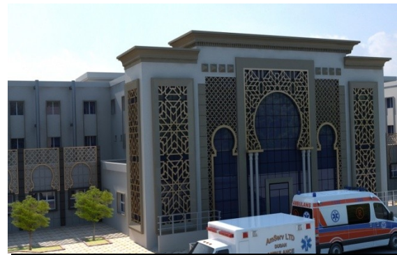
Figure 33: Hôpital 240 lit. Djelfa Source: auteur
