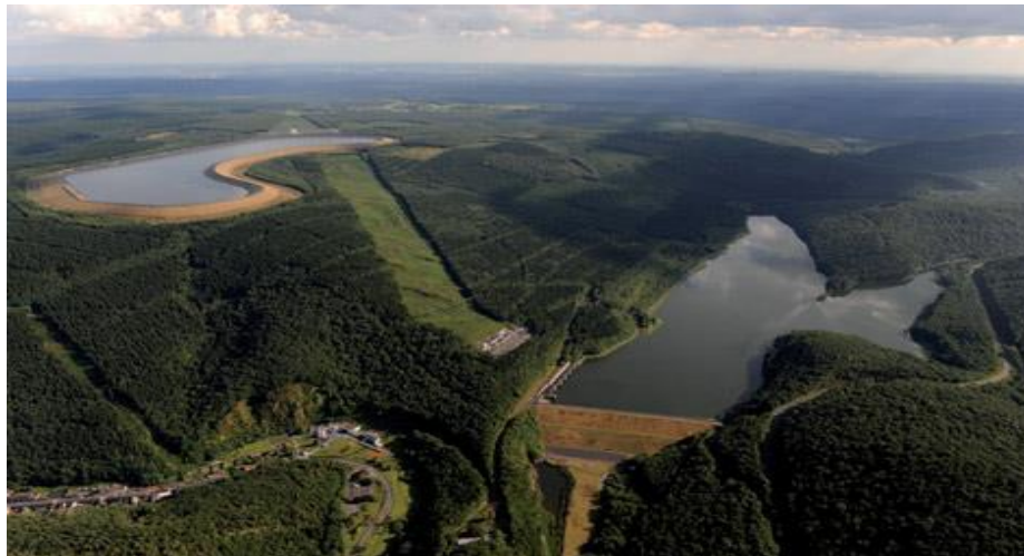
Fig I.2 View of the two reservoirs at the energy storage station
