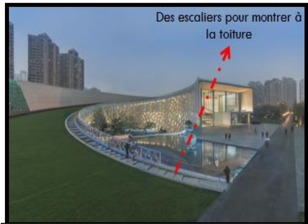
Figure II.21: toiture du musée Source: Google earth
