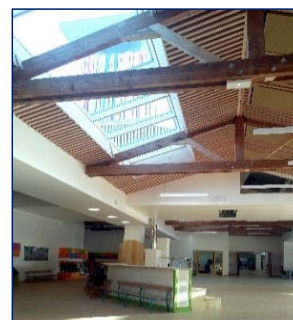
Figure 45: espace de circulation. Source : batirama.com
