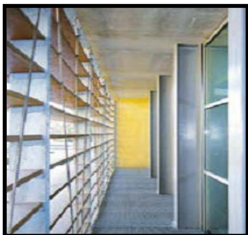
Figure 66 : Passerelle technique [source : http://www.atlas_des_colleges.com ]
