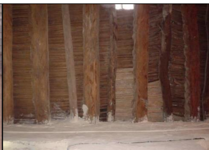
Photo 8 : planché roseaux (palmiers)
