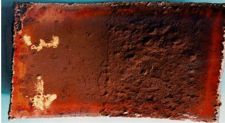
Figure III-1: Internal corrosion of a crude oil pipeline (Source http://www.corrosioncost.com/pdf/gasliquid.pdf )
