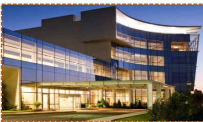
Figure I 42: Accès public principal [Source : https://www.archdaily.com ].
