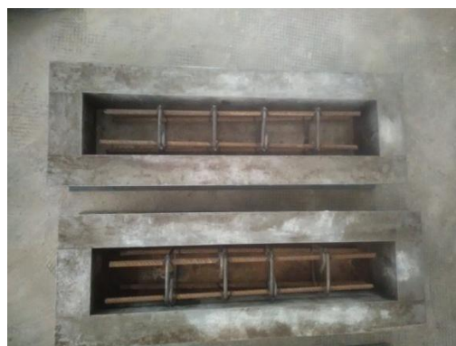
Figure II.12: Ferrailage des poutres 10x10x50 cm.
