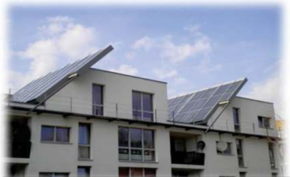
Photo 17: les panneaux photovoltaïques Source : http://www.pizzatravel.com.ua/eng/germany/9/kronsberg_district_in_hannover
