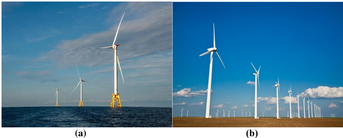
Figure I.6 : Wind Park Types : (a) Offshore [12], (b) Onshore [7].
