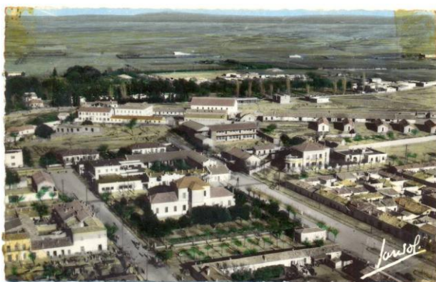
Figure 51: Djelfa, vue aérienne Source : http://www.titteri.org/v_djelfa.htm
