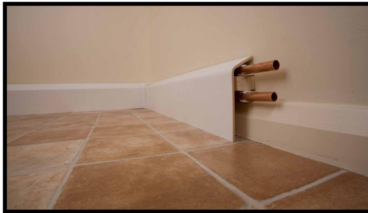
Figure 164: dissimulation des tuyaux de chauffage Source :www. google.com
