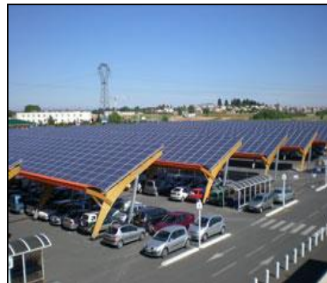
Figure IV. 11 Ombrière photovoltaïque de parking. Source: http://www.sunvie.eu/ombriere-photovoltaïque-exemple-saint-aunes.html
