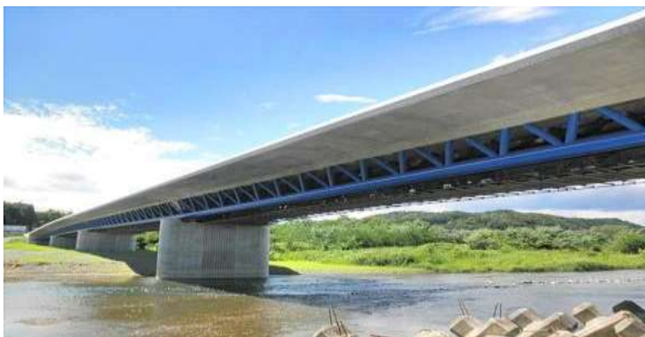
Figure I. 9 : Nagata bridge, Japan
