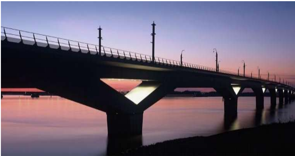
Figure I. 7 : Bridge HST, Hollandsch Diep 1998-2006
