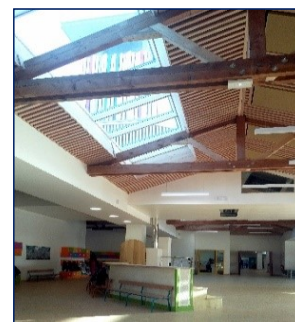
Figure 45: espace de circulation. Source : batirama.com
