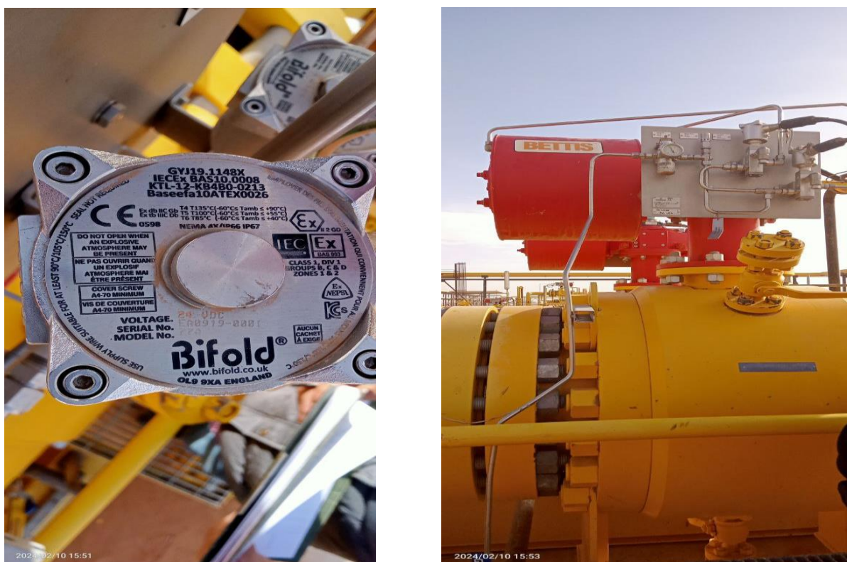
Figure 23: Electro vanne ouverture/fermeture XY420-B
