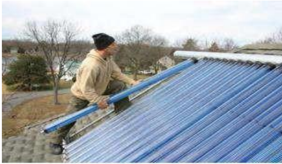
Figure II. 5: tubes under a vacuum installed in a roof.
