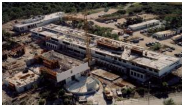
Figure 7: image montre la phase de construction
