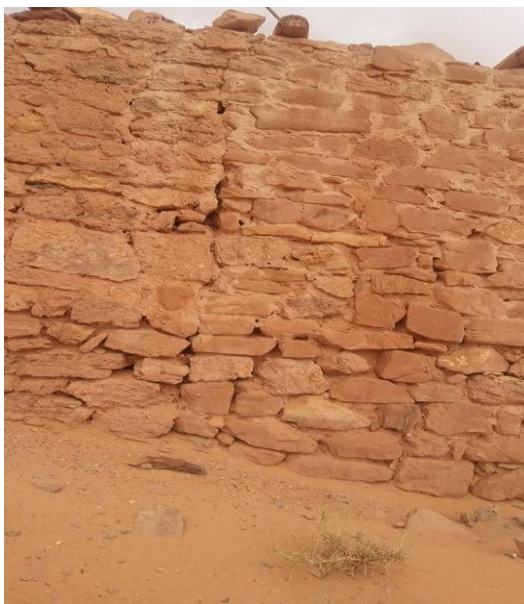
Fig. III.A..44 mur fissuré
