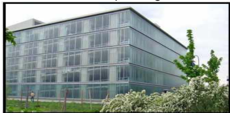
Photo 01: parkings a niveaux
