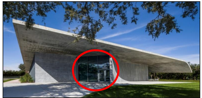
Figure 8: Entrée principale Source : https://www.archdaily.com
