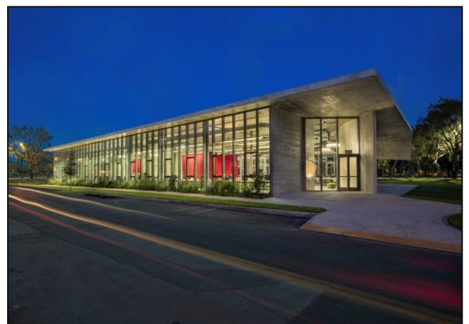
Figure 13: Entrée principale Source : https://www.archdaily.com
