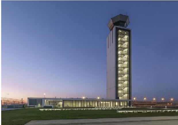
Figure A.20 : O'Hare South control Tower
