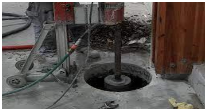
Figure II-10 : carottage
