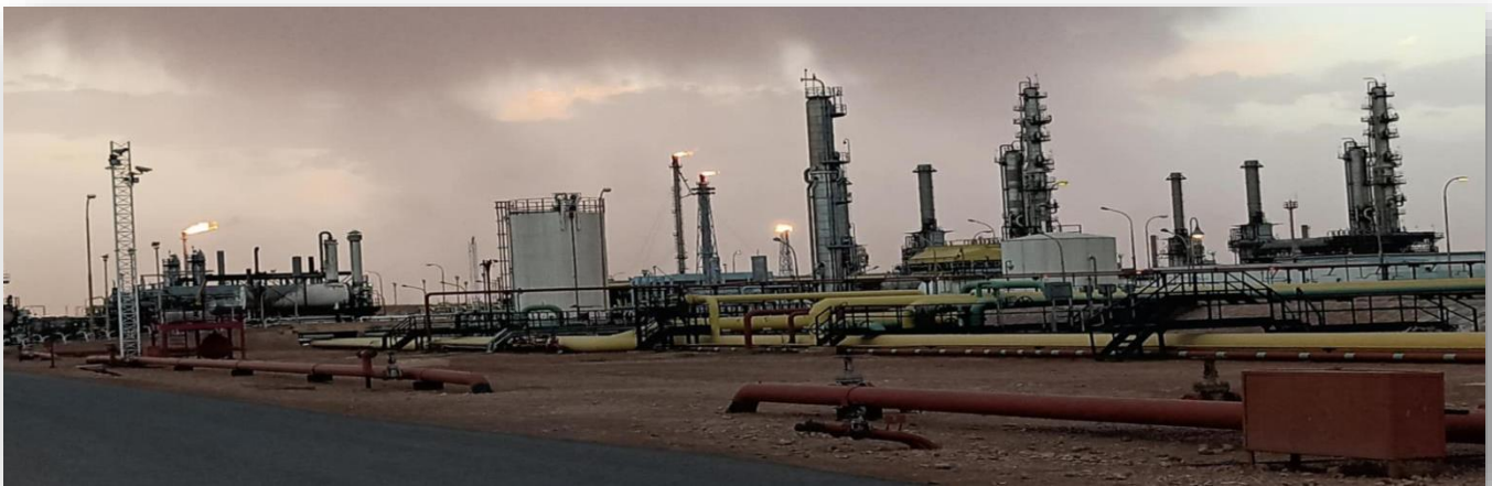
Figure 10: Module processing plant (MPP0).
