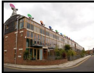
Figure III.12 : façade BDZ (la source : Google image)
