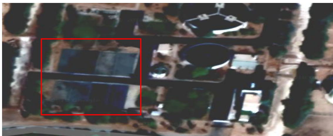
Figure 11: Image satellite des lits de séchage– STEP HASSI R'MEL (Google Earth, 2018).
