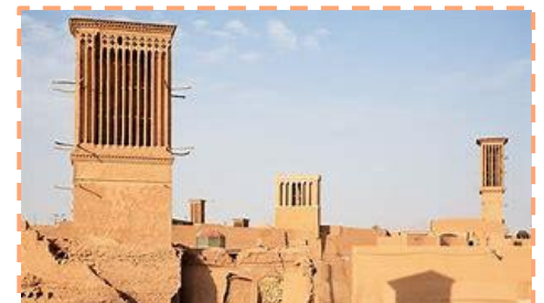
Figure 17 : Tour à vent Source : https://www.bing.com/images/search 23/07/2022 18:20
