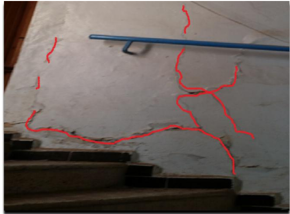
Figure III.10. Fissuration des escaliers
