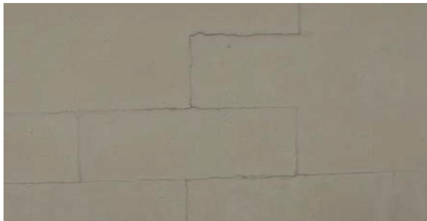
Figure II.4 : Microfissures
