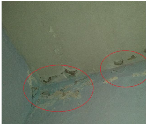
Figure III.10. Fissuration des escaliers
