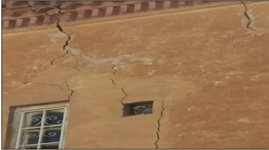
Figure III.1. Fissure façade.
