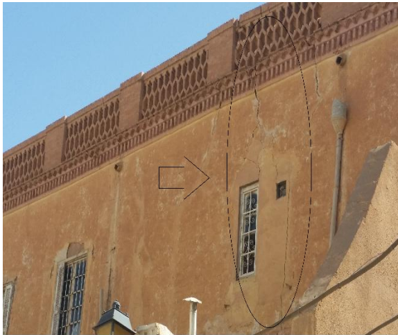
Figure III.18. Fissure profond
