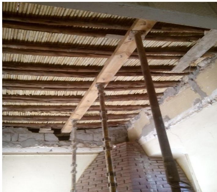
Figure III.24. Flexion du plancher
