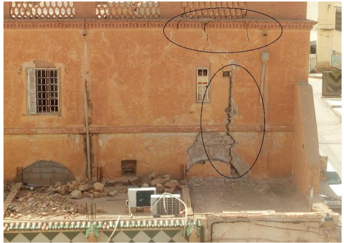
Figure III.19. Fissure verticale
