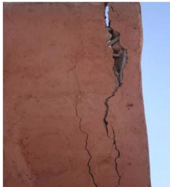
Figure II.2 : Fissure [2]
