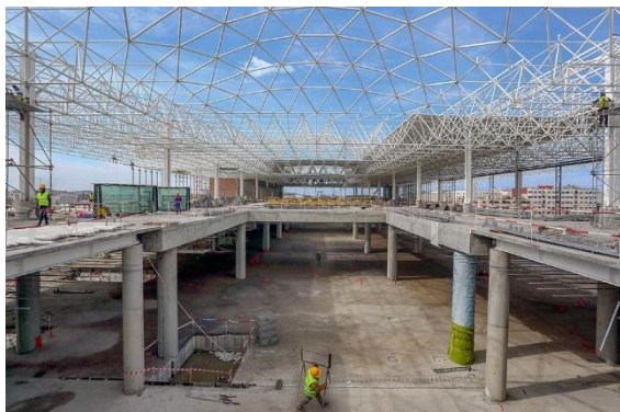
FIGURE 46:STRUCTURE DE GARE.
