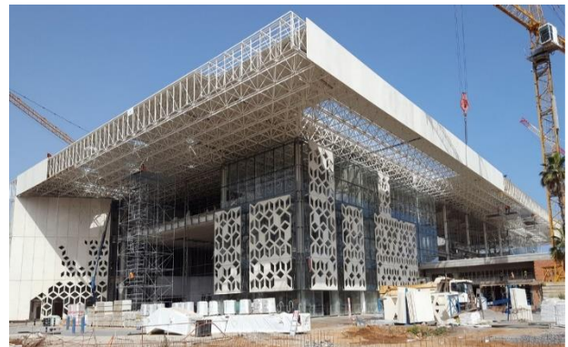
FIGURE 47:STRUCTURE DE GARE.
