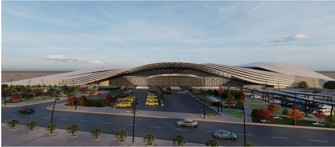
FIGURE 33 :LA FAÇADE PRINCIPALE.
