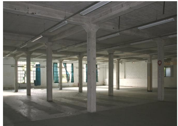
Figure V-1 : Structure poteaux-poutres.
