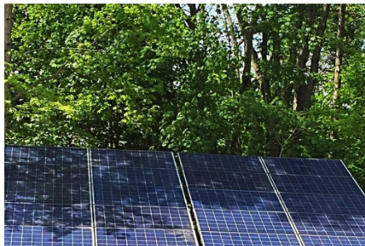
Figure 2.14: Partial shading
