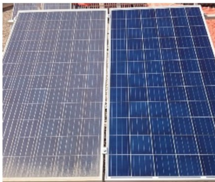
Figure 2.15: Dust impact on solar panel
