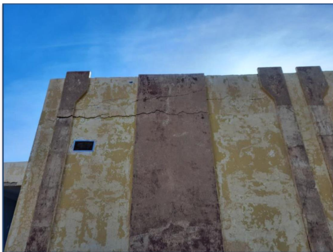
Figure II.21 : Fissures horizontales [44]
