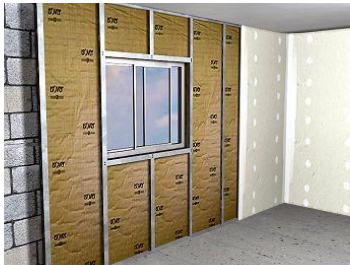
Figure II. 16: application d'une isolation interne
