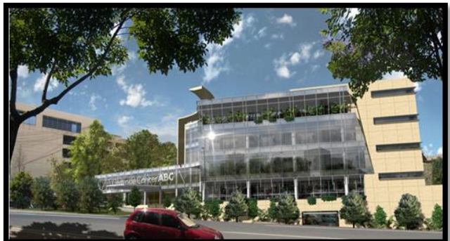
Figure 116 : Façade center anti cancer, Source : https://www.archdaily.com/161040/abc-cancer-center-hks
