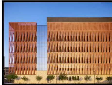
Figure 107 : façade center anti cancer Source : Arch Daily
