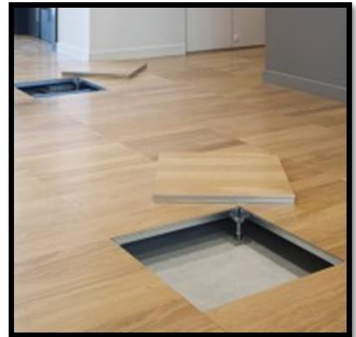
Figure 274:Le Plancher technique
