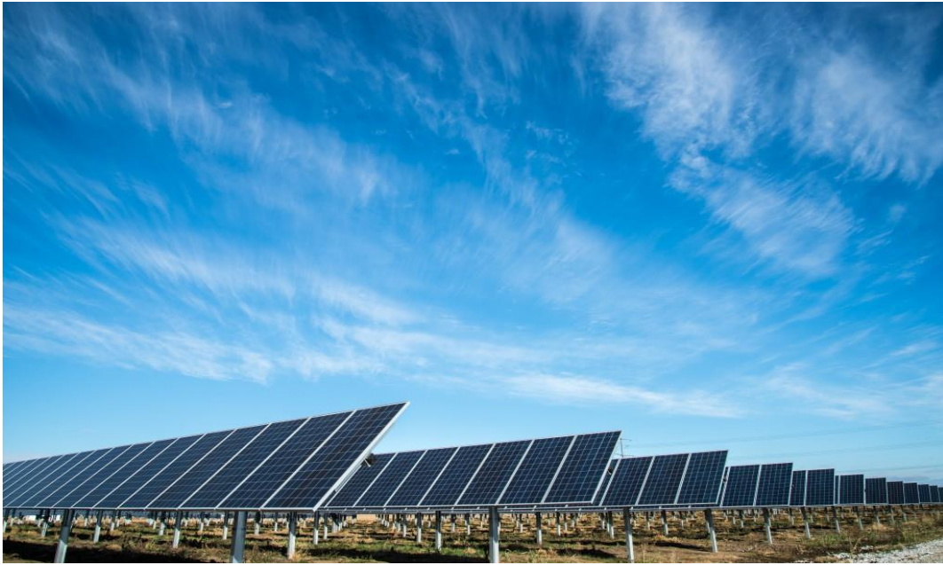
FIGURE I.10 – les plaques photovoltaïques
