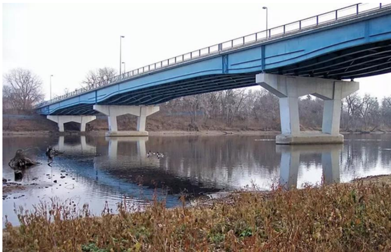
Figure 40. Continuous Beam (Bridge).
