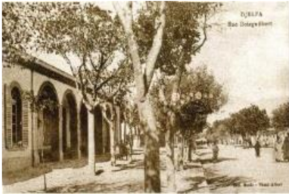
Figure 31: Rue Boisguilbert. Source : www.djelfa.org .
