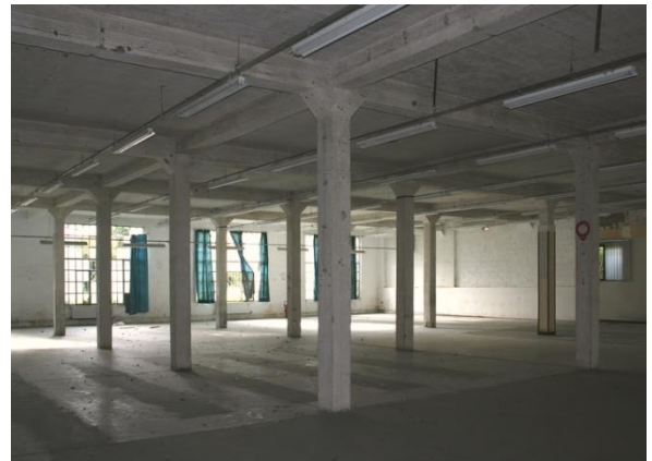
Figure V-1 : Structure poteaux-poutres.
