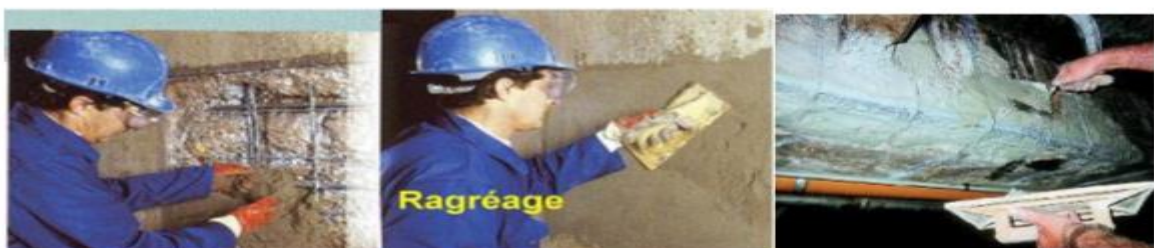
Figure II.18: Application manuelle de mortier.
