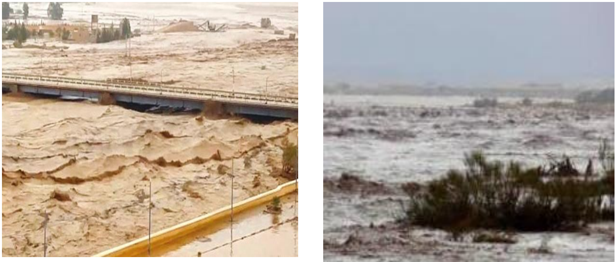
Figure 13: Inondation de barrage Tajmoute (Crues 2016 et 2018).(Bouhamam.A,2016)
