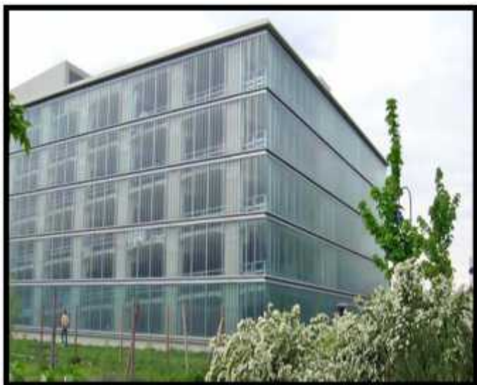
Photo 04: parkings a niveaux
