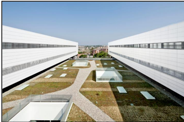
Figure 82 : toiture jardin. Source: https://www.archdaily.com/405281/sant-joan-de-reus-university-hospital-pich-aguilera-architects-corea-and-moran-arquitectura
