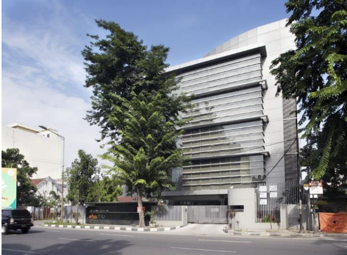
Figure 41: Façade principale. Source : https://www.archdaily.com/76805/erha-medan-hmp-architects
