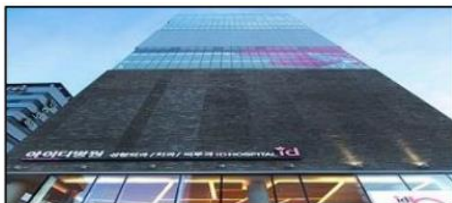
Figure 26: entree principal. https://www.archdaily.com/887840/id-hospital-dongjin-kim-plus-leau-design
