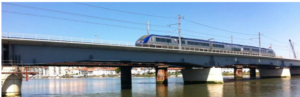
Figure I.2. Pont rail mixte.
