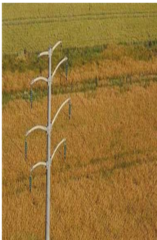
Figure I-8: Pylône Muguet
