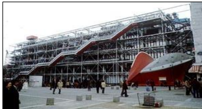
Figure N 28 : Pompidou, France.
