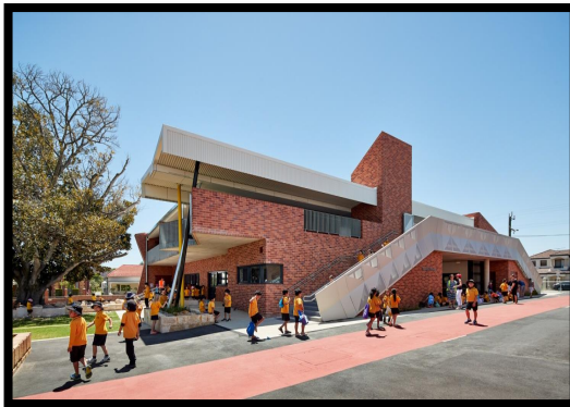
Figure 1.1 : Primary School (sandri house) Source: www.archdahily.com
