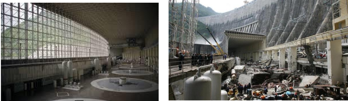
Figure 16. Sayano-Shushenskaya power station accident before and after.
