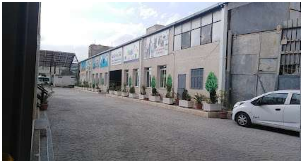
Figure 1 national waste agency headquarters (Djeddou, 2021)
