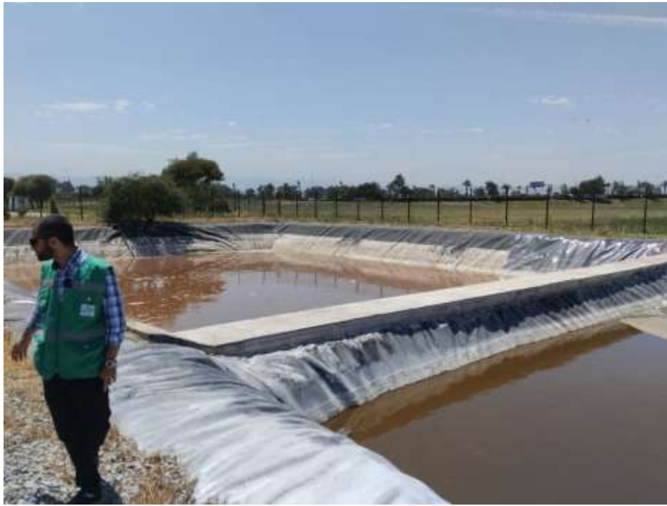
Figure 36 Leachate basins (Benaissa, 2023)
