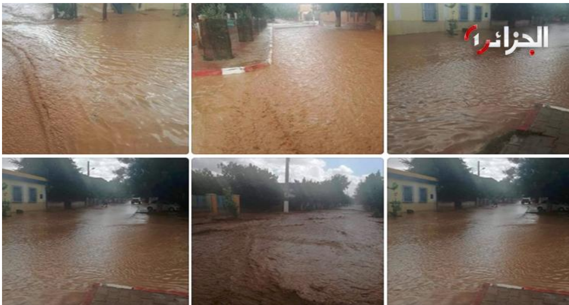
Figure 19. Inondation de Batna22/08/ 2018(source : internet)
